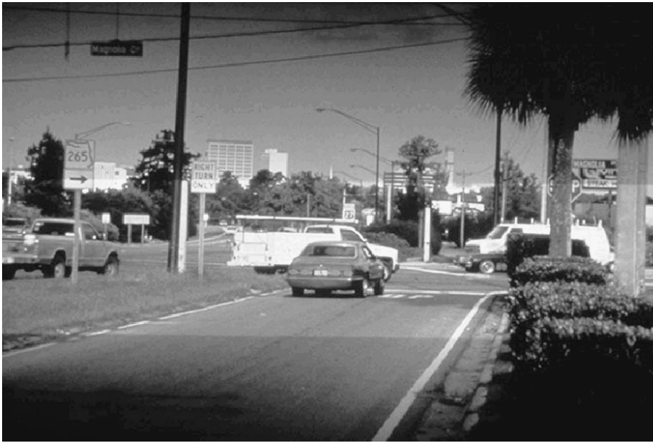
FIGURE 10-30 Confusing intersection where frontage road connects too close to a major side street.
